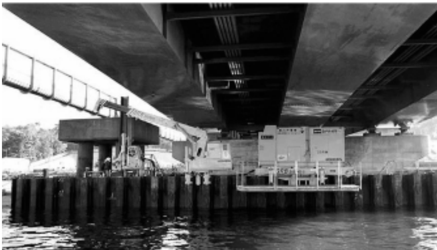
Figure 11 Piling work under the bridge
