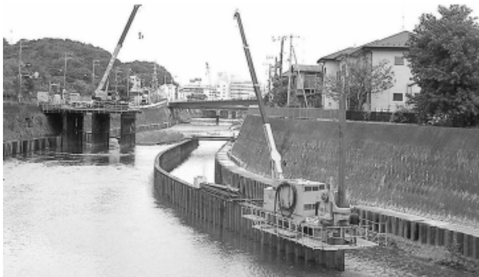
Figure 12 Piling work along the river
