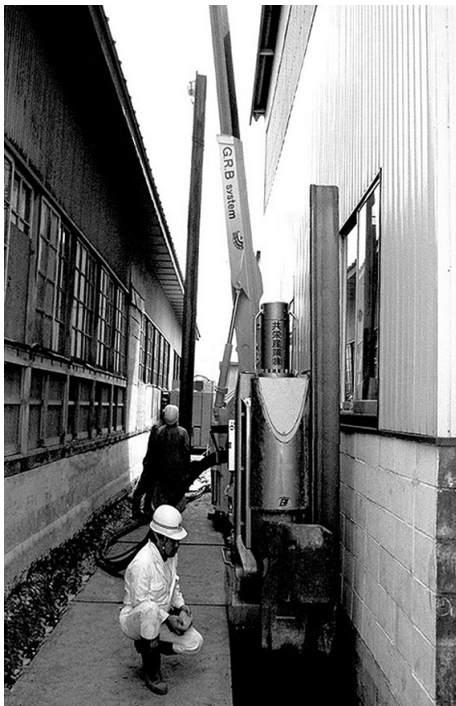
Figure 10 Piling work at the marginal area
