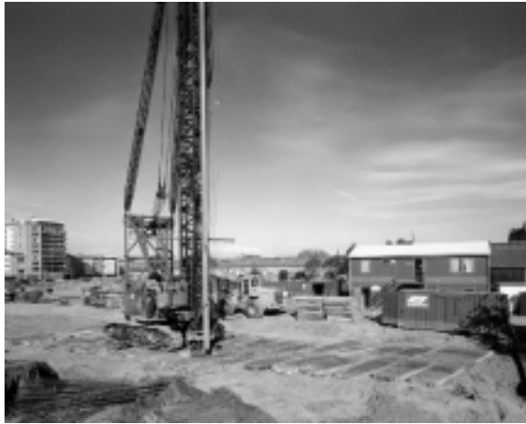
Figure 3. Overview of the building site in Delft.
