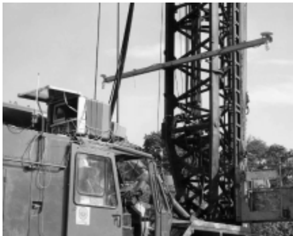
Figure 4 Equipment on the piling rig
