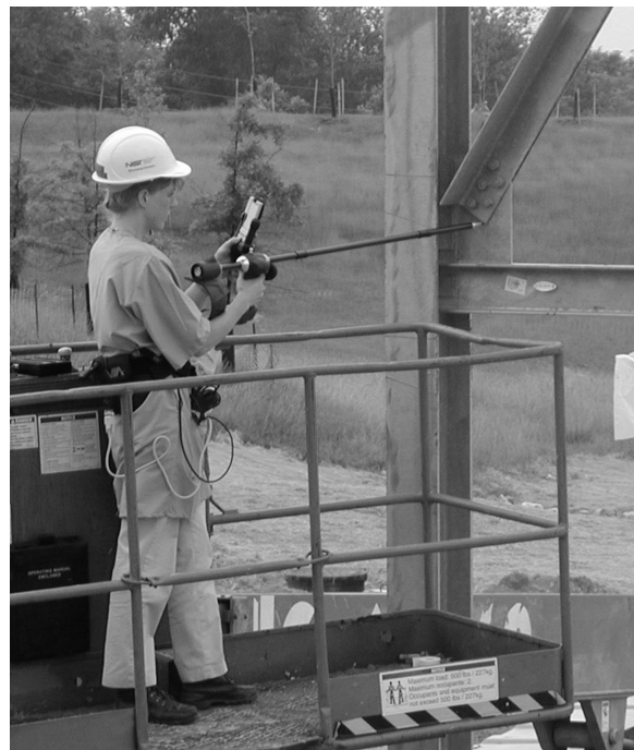
Figure 2. Field operator collecting fiducial point coordinate data with the Vulcan receiving tool integrated with the VIA belt-wearable computer and bar code scanner. A manlift was used to facilitate data collection once the steel tower was erected and installed in its final location.
