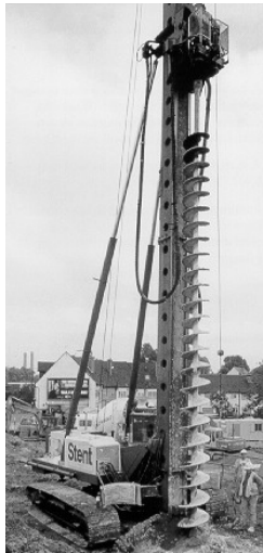
Figure 1. CFA Piling Rig.
