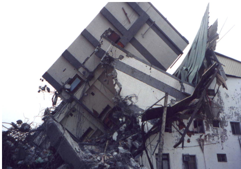
Picture 1. The Da-li-wang-chao building in the city of Taichung collapsed and hit the adjacent building (Photo credit: Chung-Wei Chen, Dept. of Civil Engineering, National Taipei Univ. of Technology)
