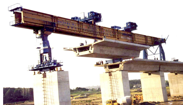
Figure 2. The girder forwarding by gantry Launcher operate in Pyung-Taeck, Korea HSR Lot 3
