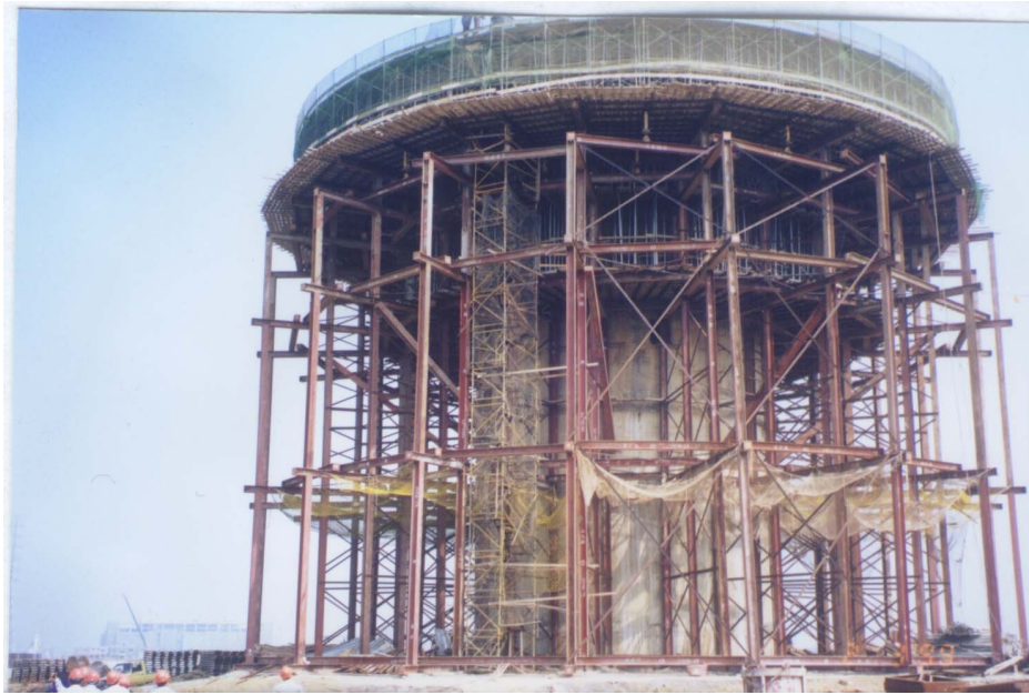
Figure 2. Conventional scaffolding system
