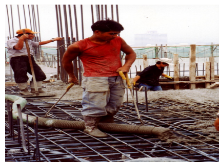
Figure 1. Concrete Placing Activity
