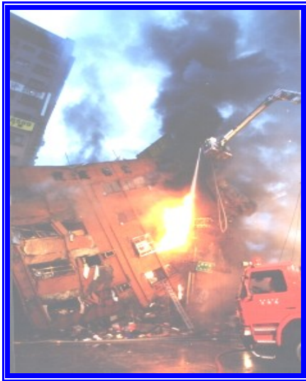
Picture 1. The collapsed Dong-Xing building.
