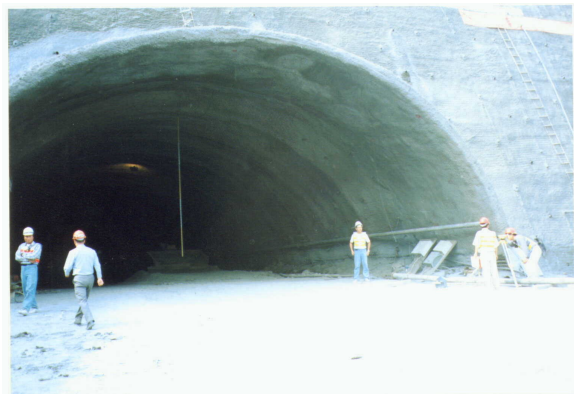
Figure 5. The conventional displacement monitoring methods (Roof-leveling)
