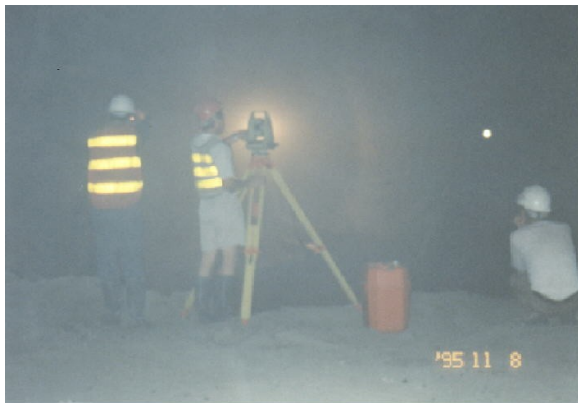
Figure 7. The 3D-optical monitoring (Shotcrete)
