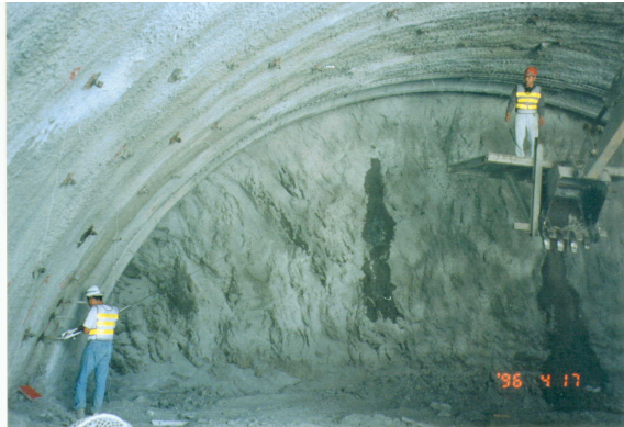
Figure 1. The conventional displacement monitoring methods (Convergence)
