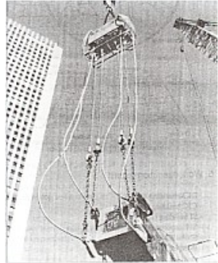
Fig. 5 Radio controlled steel beam handling robot (courtesy: Shimizu Corp.)
