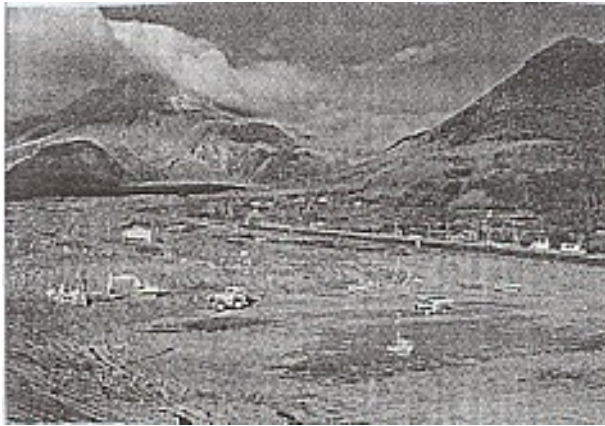
Fig3. A case of remote controlled un-manned earth work
