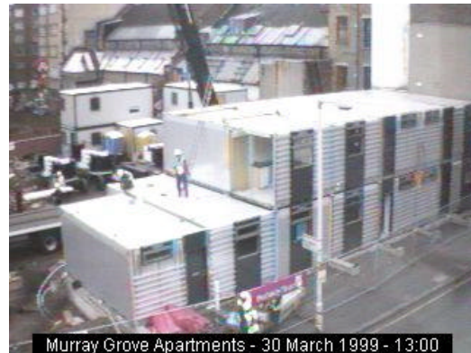
Fig 4. Murray Grove modular housing project under construction.
