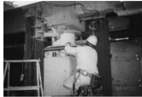
Photograph. 7 Handling a laminated rubber bearing
