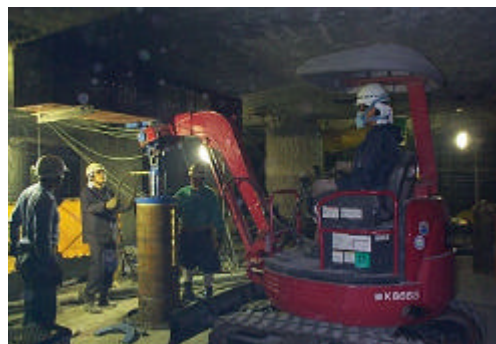
Photograph. 8 Pressing-in steel pipe pile
