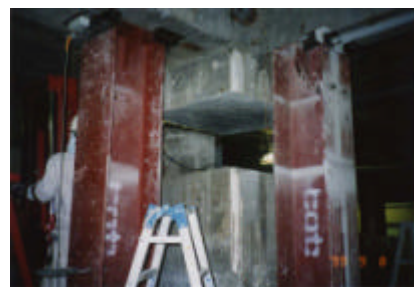
Photograph. 3 After the column cutting ends
