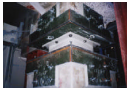
Photograph. 4 After the laminated rubber bearing installation ends
