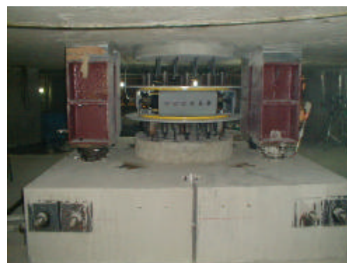
Photograph. 9 Status that laminated rubber bearing is fixed
