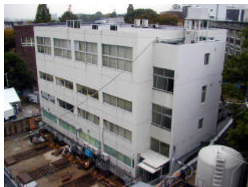
Photograph. 10 Building B panorama
