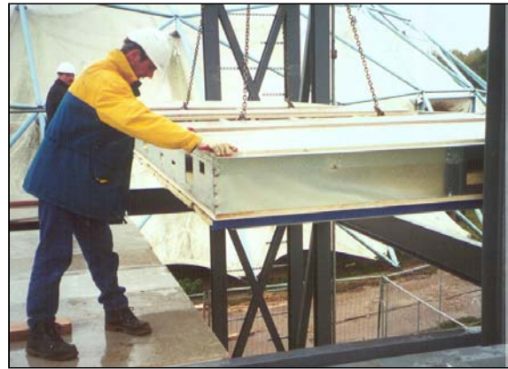
Figure 2. Assembling the floor panels.
