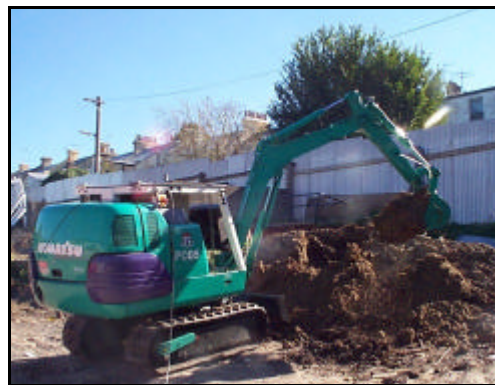
Figure 3. University of Sidney's automated excavator.
