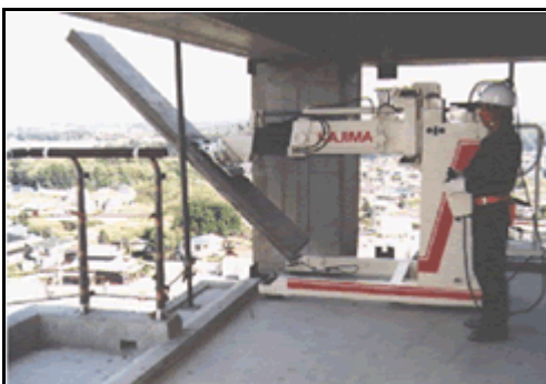
Figure 5. Kajima’s interior wall assembly robot.
