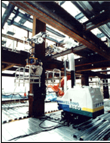
Figure 8. WR mobile robot for column welding
