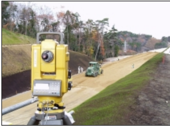
Photo 4. Job site work of 3D-MC grader
