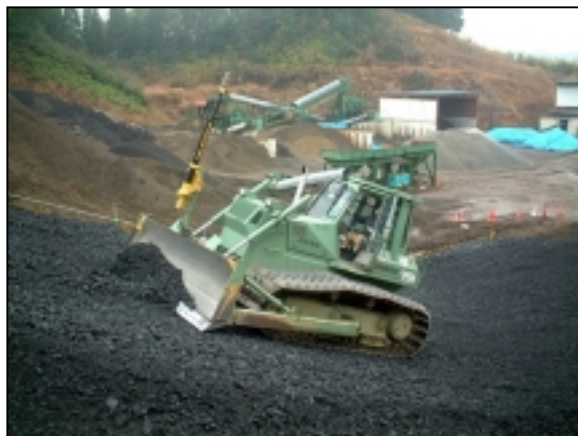
Photo 5. 3D-MC bull-dozer at dam construction
