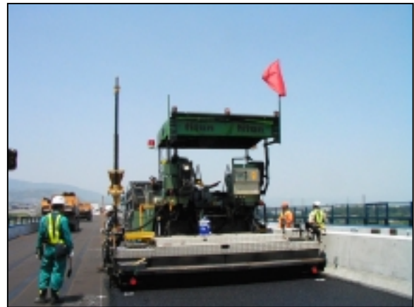
Photo 6. Paving work of 3D-MC asphalt finisher
