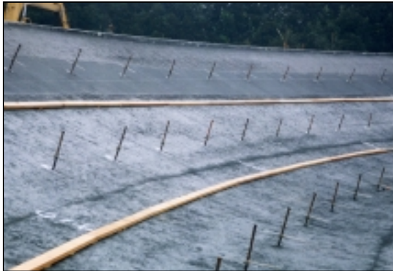
Photo 1. Stakes for machine control set on slope
