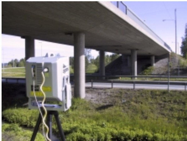
Figure 6. Measurement of an old bridge - Tampere.
