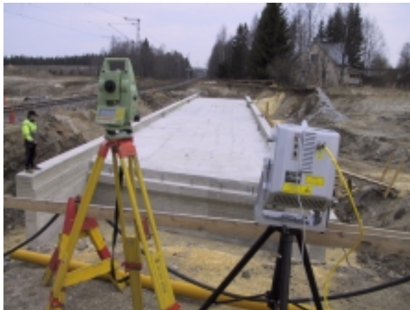
Figure 5. Controlling the accuracy of concrete bridge structure - Suonenjoki.
