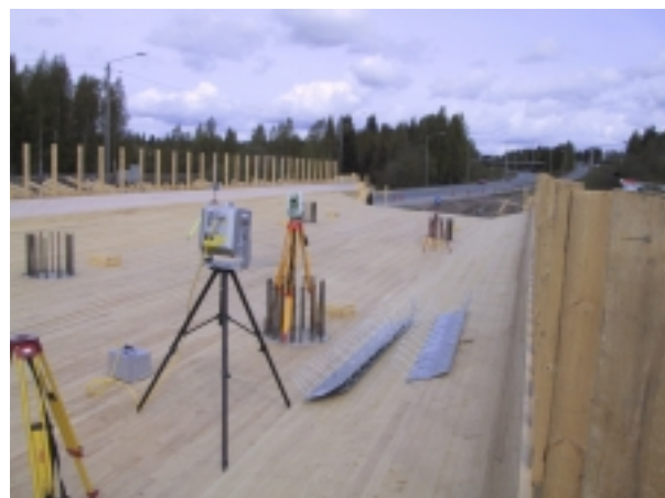
Figure 4. Controlling the accuracy of bridge mould by Cyrax laser scanner - Varkaus.
