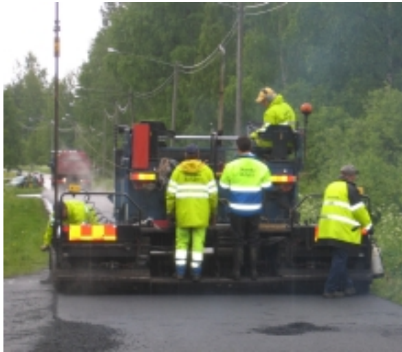
Figure 5. Testing the first Finnish 3-D machine control system for asphalt spreader – Summer 2004 Finland.
