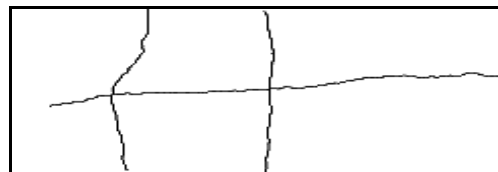
Figure 10. Extracted crack of indoor wall
