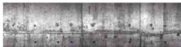
Figure 11. Image of subway inner wall
