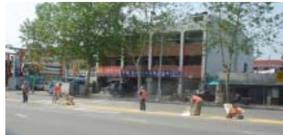
Figure 1. Working field for road marking removing
