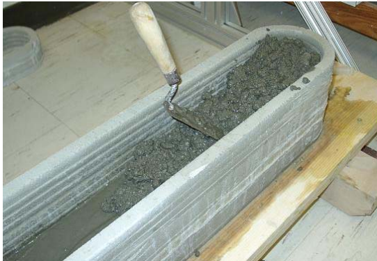
Figure 9. Pouring concrete in layer by layer
