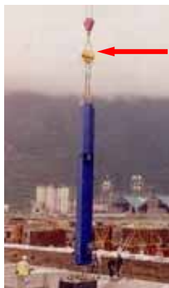
Figure 2. Setting up a vertical beam
