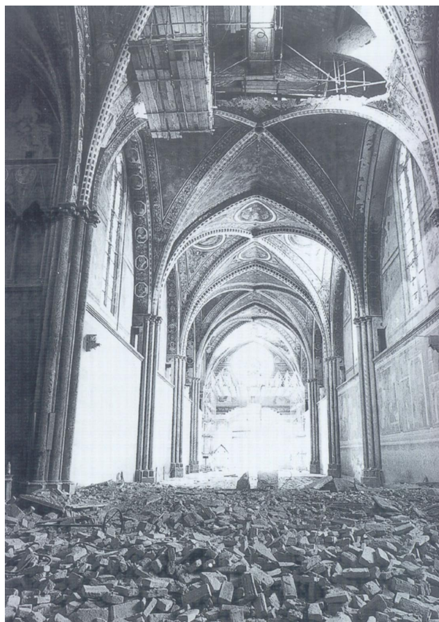
Fig. 1. The interior of the Upper Church of St. Francis in Assisi after the earthquake in 1997 [2].
