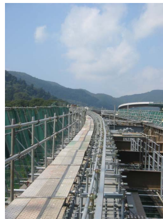
Fig. 9. Rail installation
