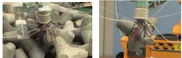
Photo.13 Tightening. Photo.14 Block lifting
