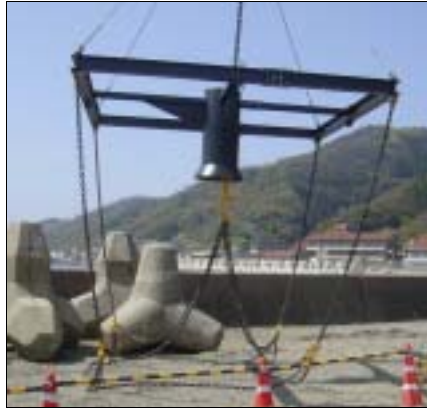
Photo.22 Block transfer device
