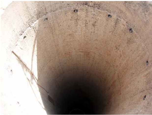
Figure 15: Cleaned concrete surface
