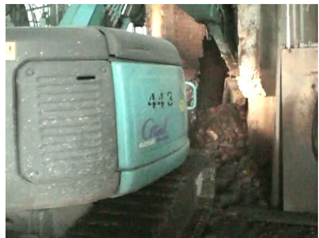
Figure 14: Removal of bricks by a backhoe
