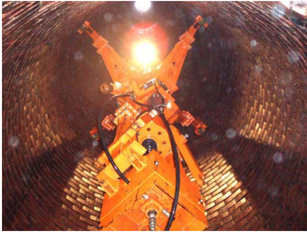
Figure 11: Cleaned brick surface viewed upward from the chimney bottom
