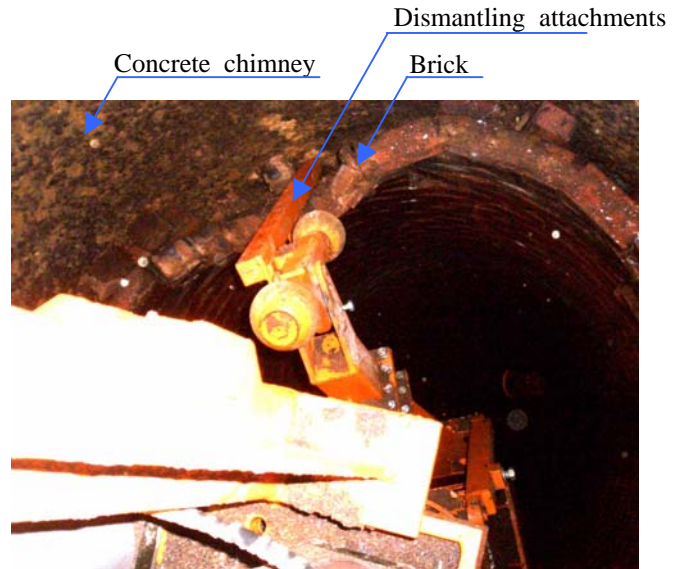
Figure 13: Brick dismantling
