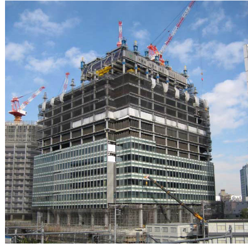
Photo 2. Building of Project O under Construction
