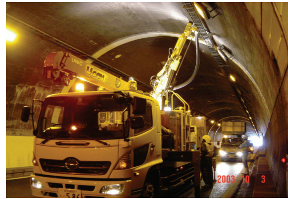
Photograph 3 Checking for voids behind lining by drilling holes 5)
