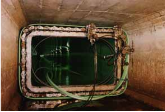
Fig.-10 : View of existing pipeline
