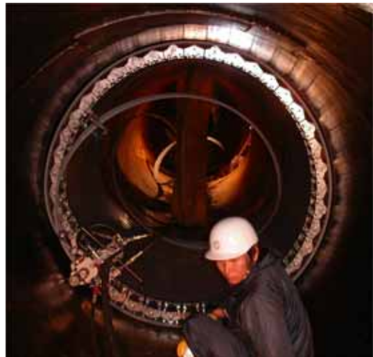
Fig.-14 : Status of Simultaneous Liner Installation and Grouting
