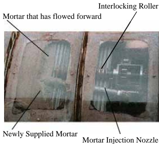
Fig.-7 : Simultaneous Liner Forming and Grouting - 2
