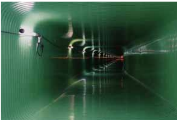
Fig.-13 : Liner after Rehabilitation
