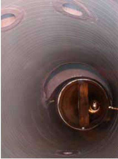
Fig.-15 : Inside the Liner after Rehabilitation
