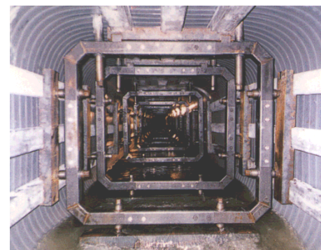
Fig.-4 : Installed Support Jacks
