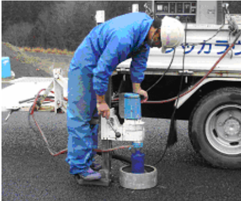
[IT-assisted construction: TS-based survey]
