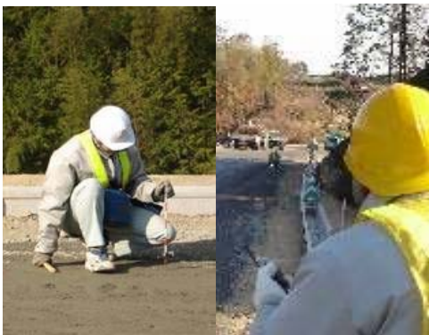
Photo 4 Comparison of layer thickness inspection
