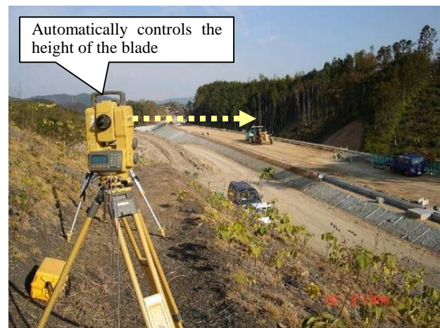
Photo 3 IT-assisted sub base shaping work
