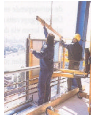
4. Wall panels are connected to the tower crane.
