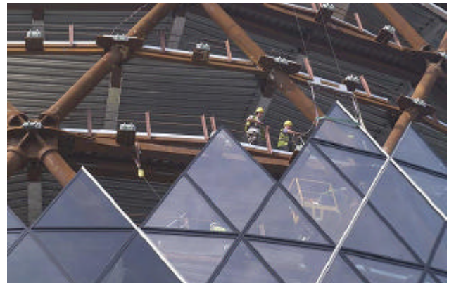
Figure 1: Curtain wall assembly can be extremely dangerous. The photo shows the assembly of the wall panels for the St. Mary Axe high-rise building in London. (Photo: Grant Smith)
