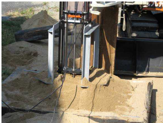
Photo-5 Cone penetration test by remotely controlled method
