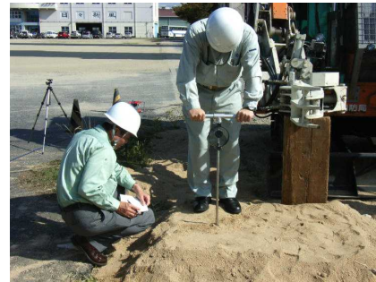
Photo-2 Portable cone penetration test by conventional method
