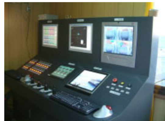
Figure 6 Remote monitoring and control panel
