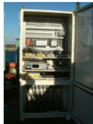
Figure 7 Wireless control panel
