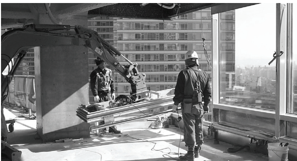
Figure 1. A mini-excavator with 1DOF mechanism
