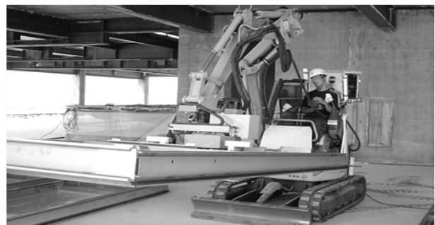
Figure 2. ASCI (Automation System for Curtain wall Installation)
