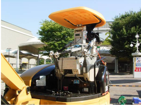
Photo-2 Remotely controlled robot mounted on backhoe
