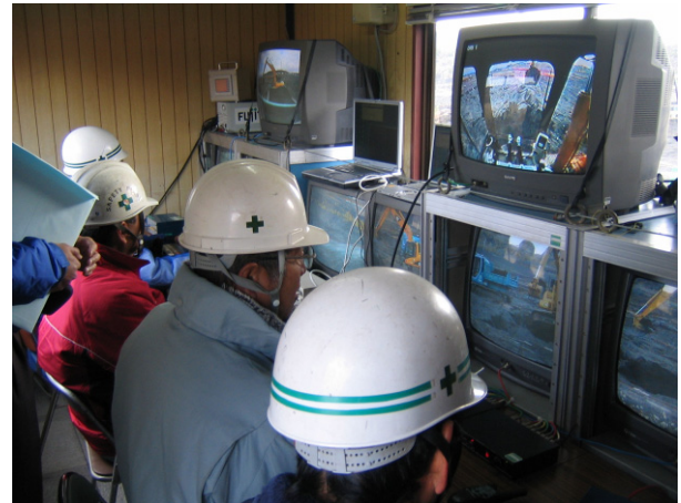
Photo-6 Remote control at operation room
