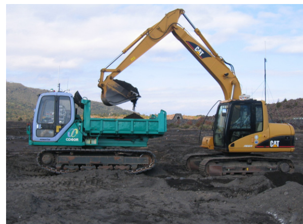
Photo-4 Excavation /loading
