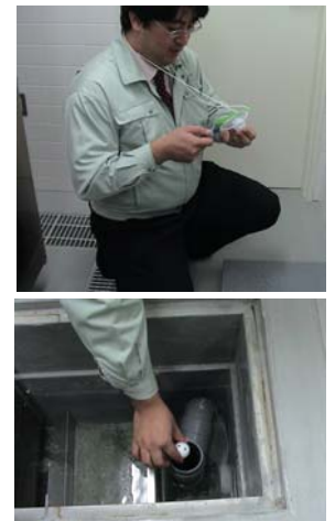
Fig.5 Operation at Starting Point
