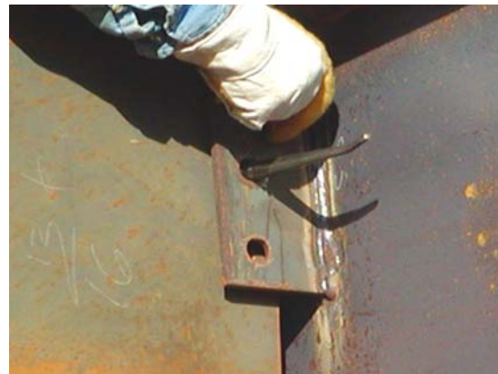
Figure 2. Using a spud wrench to align holes during initial assembly. (Source: AISC)
