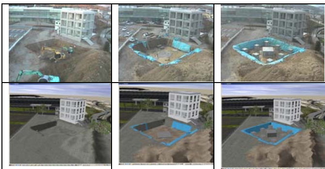
Figure 13 A photo Image and a VR Image of the ongoing construction
