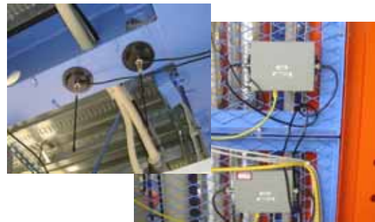
Fig.4.7 RFID Installed Inside Building
