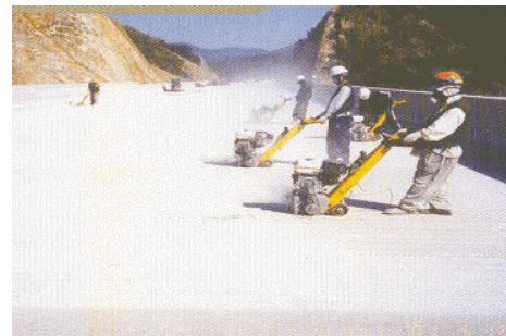
Figure 1. Manual Operation of Concrete Surface Grinding
