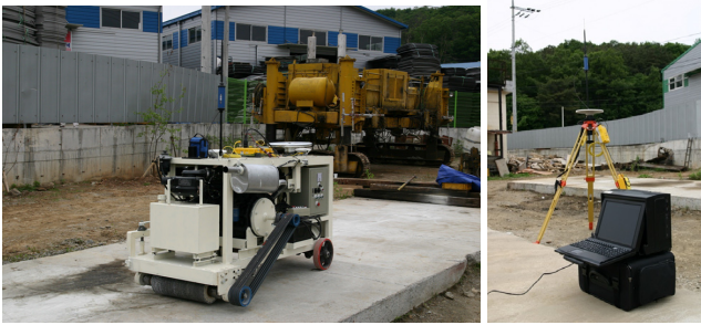
Figure 9. Concrete Surface Grinding System
