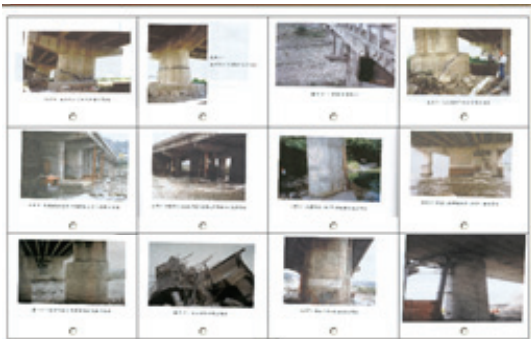
Figure 4 Photos of Historical Damaged Cases
