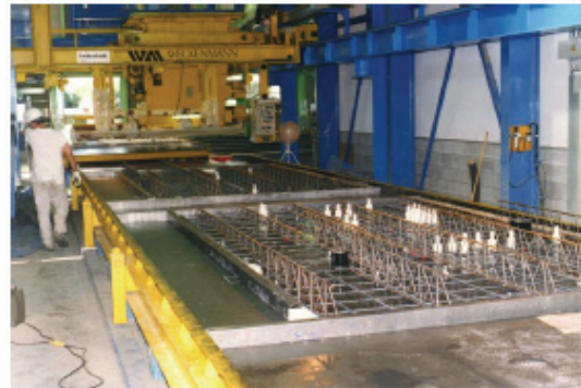
Figure 6 Pallet in concreting station
