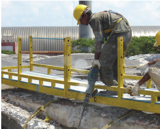
Figure 11 Demolition using Electric Chipper
