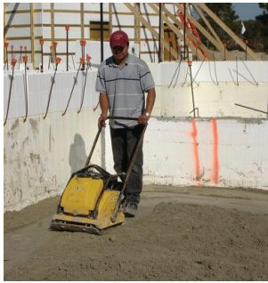
Figure 2 Compaction using Rammer
