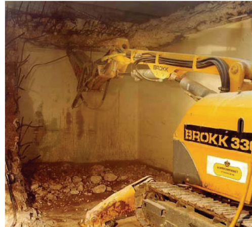
Figure 12 Demolition using Hydraulic Crusher
