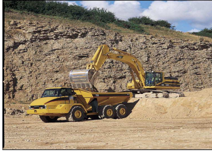
Figure 2 - Building machine group: excavator + transport means (model example)
