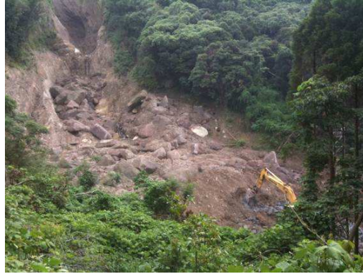
Figure 6 – Disaster Restoration Work Site (Landslide at Minamiosumi, JAPAN)
