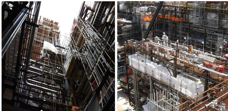
Figure 1 – Use of scaffolding in industrial construction site
