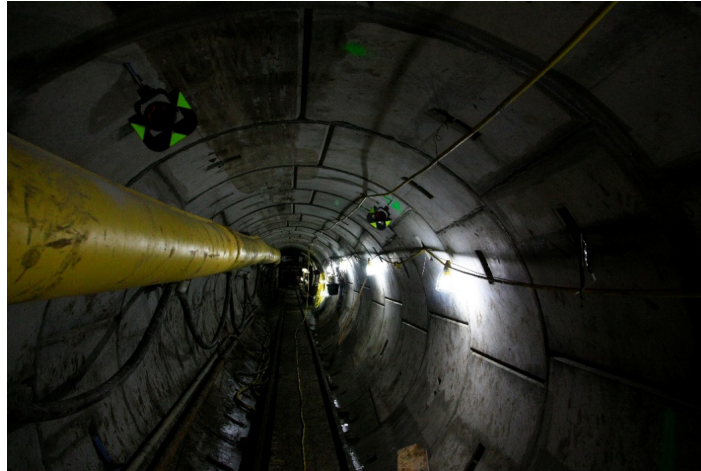
Figure 1 – Typical environment in tunnels built by TBMs
