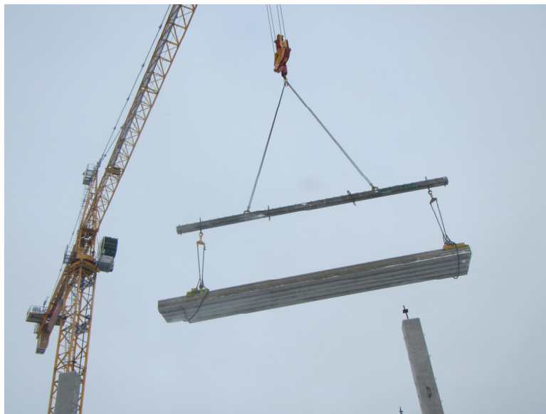
Figure 2. The studied tower crane Potain MD365 in operation.
