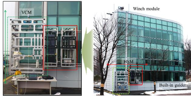
Figure 1 – System configuration
