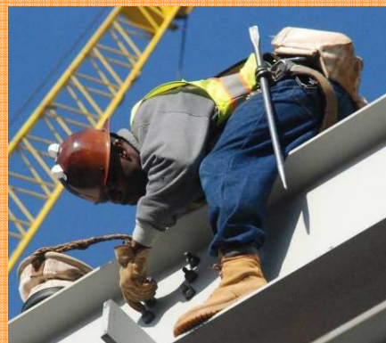
Tracking Workers for Work Zone Safety
